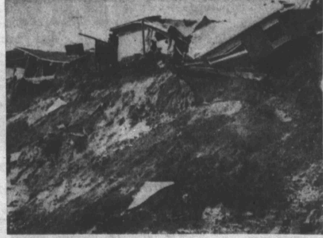
Tyler Upham home (right) lost its living room. Officials said five other homes are threatened by the slippage, which geologists say appears to be due to water seepage. It began weeks ago. (AP WIREPHOTO)
