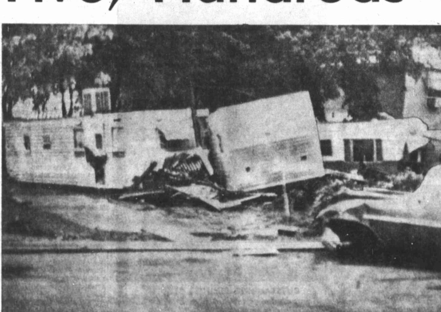
Dallas Area Flash Flood Wrecks Trailers. These trailers were torn from their foundations and piled against each other when a heavy thunderstorm sent a nearby creek surging over its banks today. Tremendous rains flooded hundreds of other persons from their homes in Dallas and a suburb to the north, Garland. (AP WIREPHOTO)
