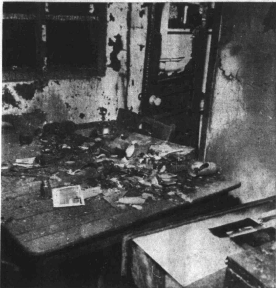
FIRE DAMAGE HEAVY INSIDE HOUSE OF TRAGEDY Near this table, the body of M. J. O'Brien, a gunshot wound in the head, was found late Sunday night by investigating officers.
