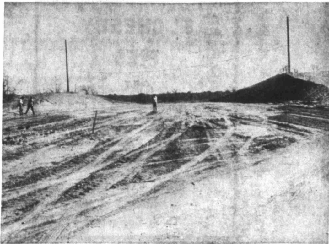
FM 700 North Construction Moves Ahead
