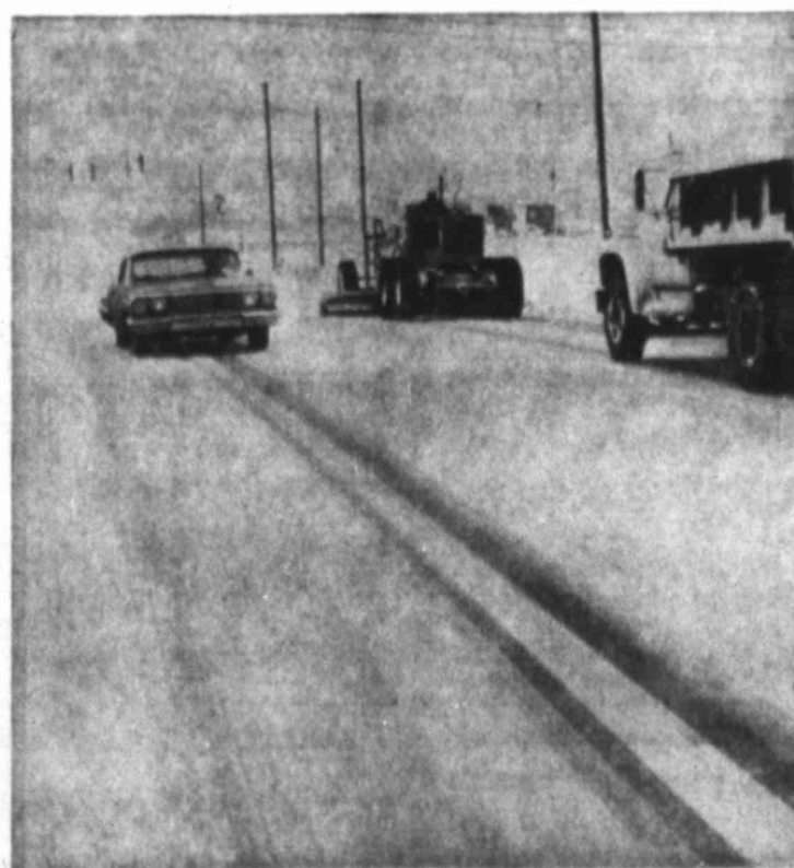
HIGHWAY CREWS AT WORK Clearing major thoroughfares
