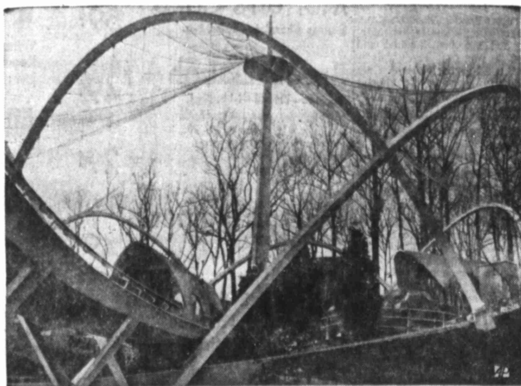
A CONFINED PATTERN — This is the flight cage for the birds of Washington's National Zoological Park. A 90-foot mast and parabolic steel arches support a vinyl-coated wire mesh that encloses the birds yet allows for fresh air and flying space.
