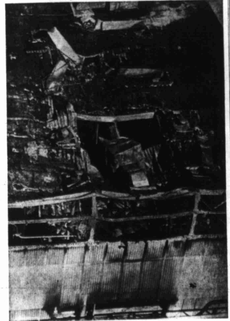
SPECTACULAR FIRE ... but refinery damage slight
