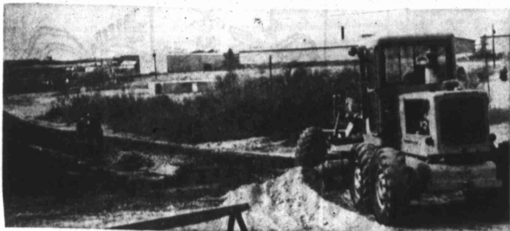
ACCESS ROAD PROVIDED ... to Lakeview School area
