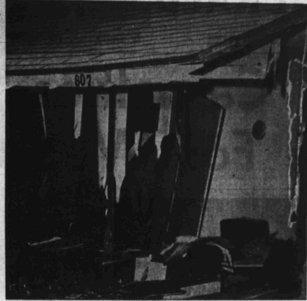
Remains Of Car-Struck Residence
