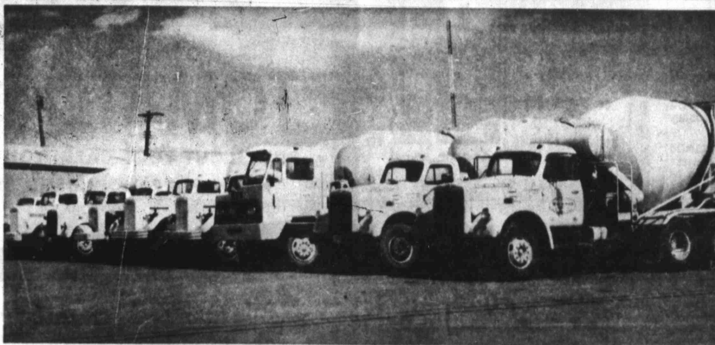
Ready-Mix Saves Many A Blistered Hand
