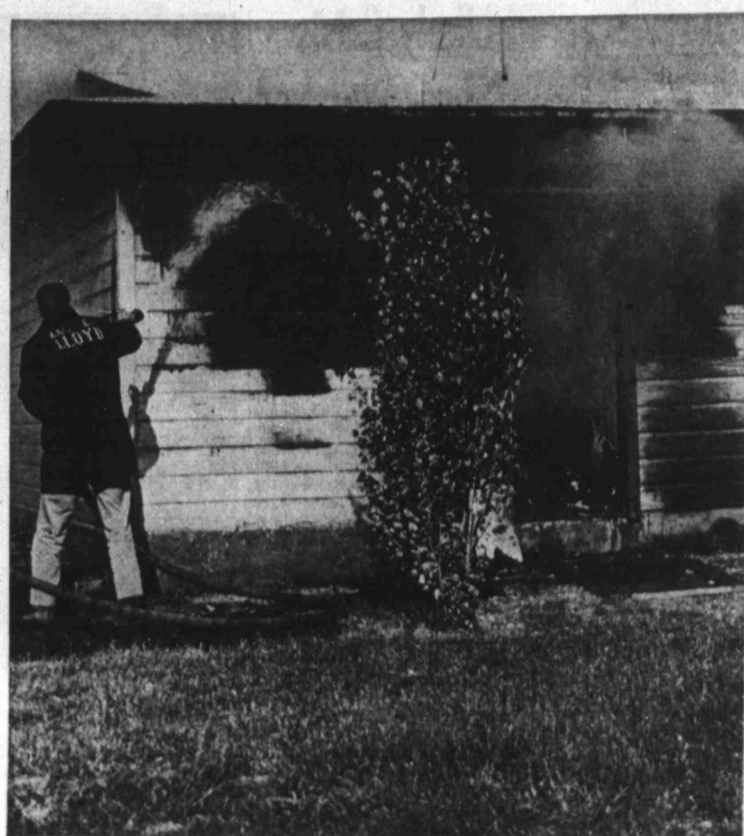
Fireman Soaks Burning Home
