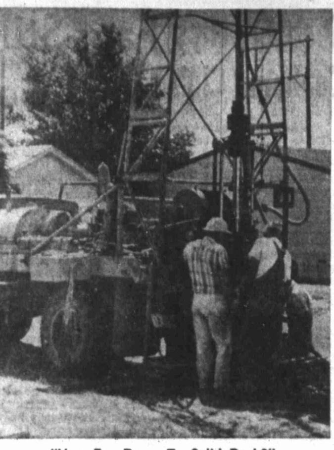
"How Far Down To Solid Rock?" Test holes drilled on post office site.
