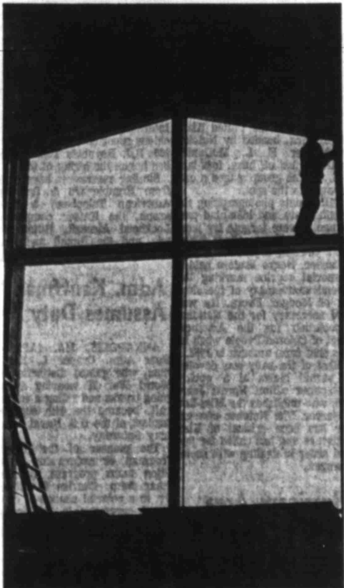
FIRST BAPTIST WORK CONTINUES Workers move inside for final months
