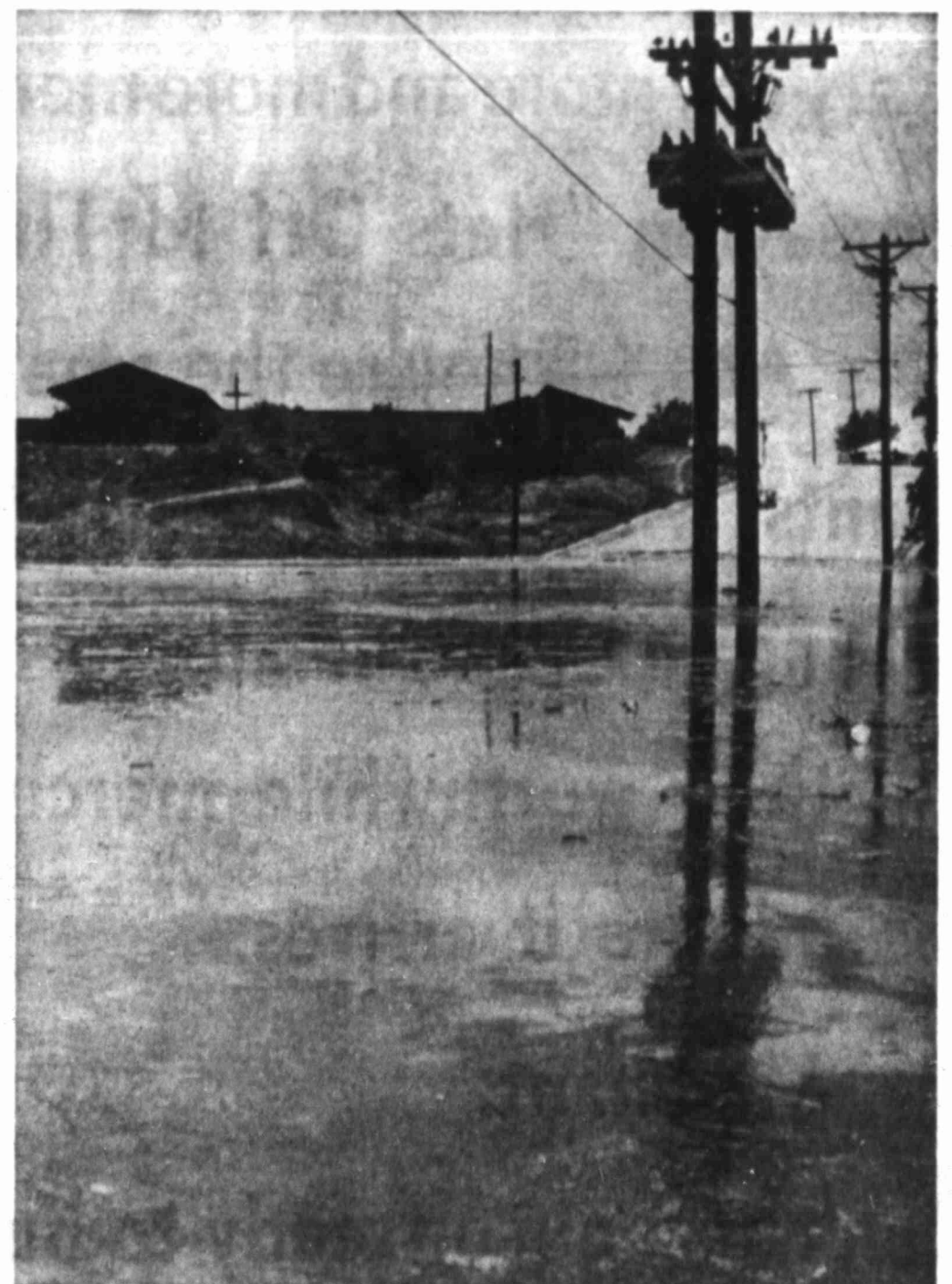
TENTH STREET FERRY Water backs over street at Birdwell Park
