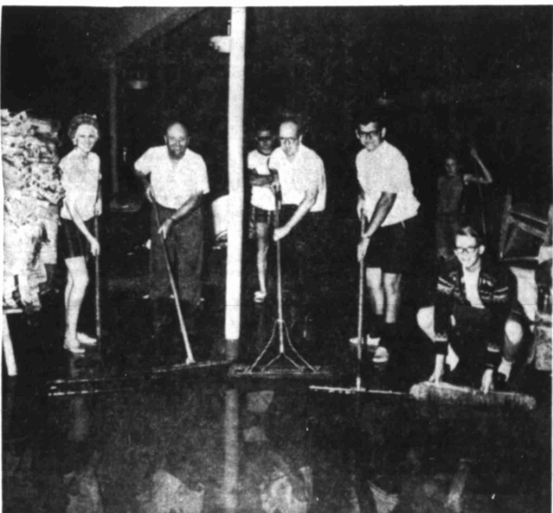
FRIENDS PITCH IN TO HELP AT ELROD'S Floor inundated as south wall collapses
