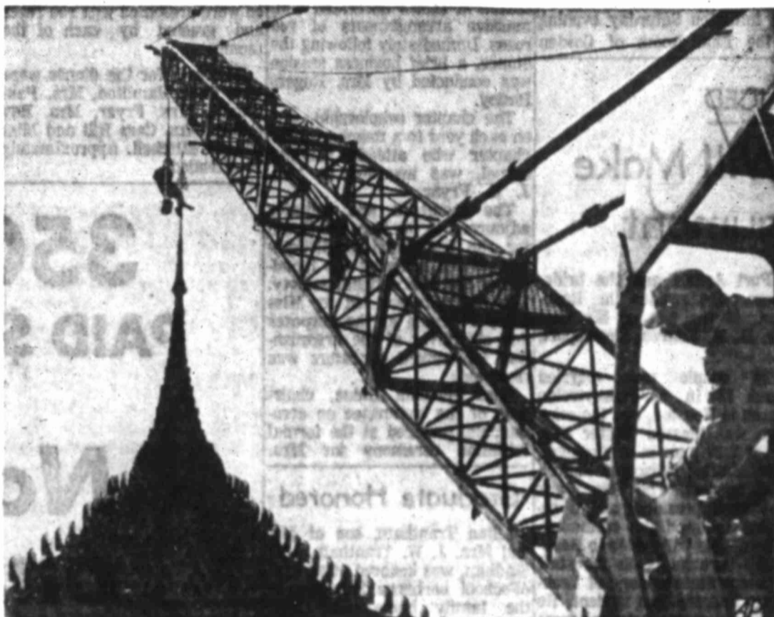
ASPIRING TO SPIRE — A painter in bosun's chair is dwarfed by the giant crane carrying him to paint the top of the spire of the Thailand Pavilion at the New York World's Fair. The exposition is readying to reopen for its second year in late April.
