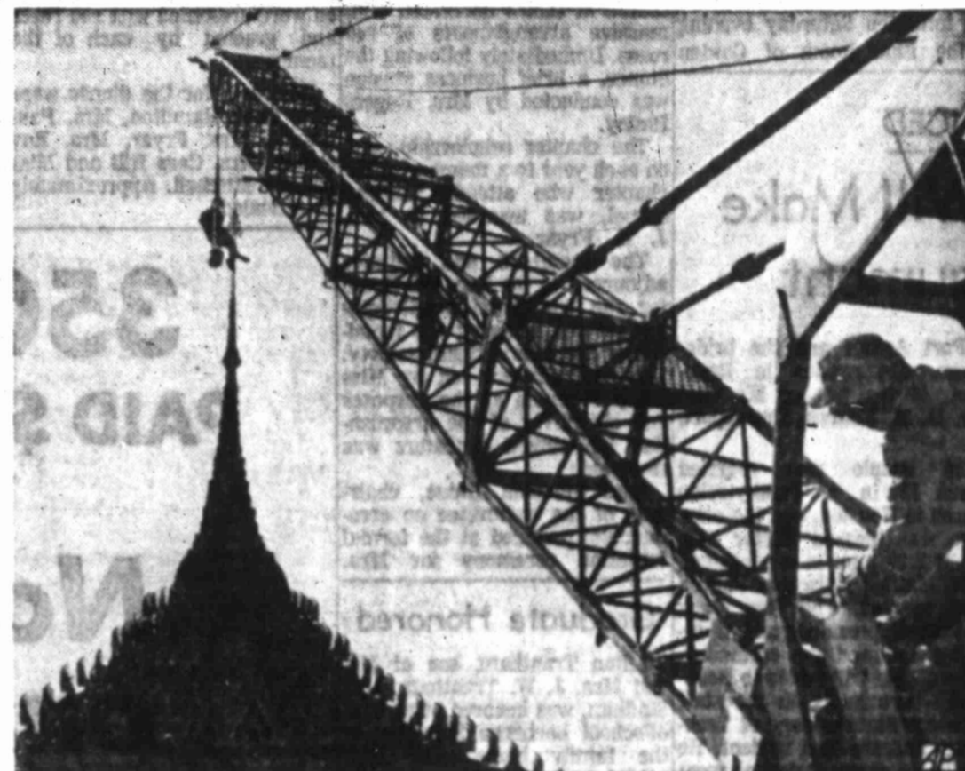
ASPIRING TO SPIRE — A painter in bosun's chair is dwarfed by the giant crane carrying him to paint the top of the spire of the Thailand Pavilion at the New York World's Fair. The exposition is readying to reopen for its second year in late April.
