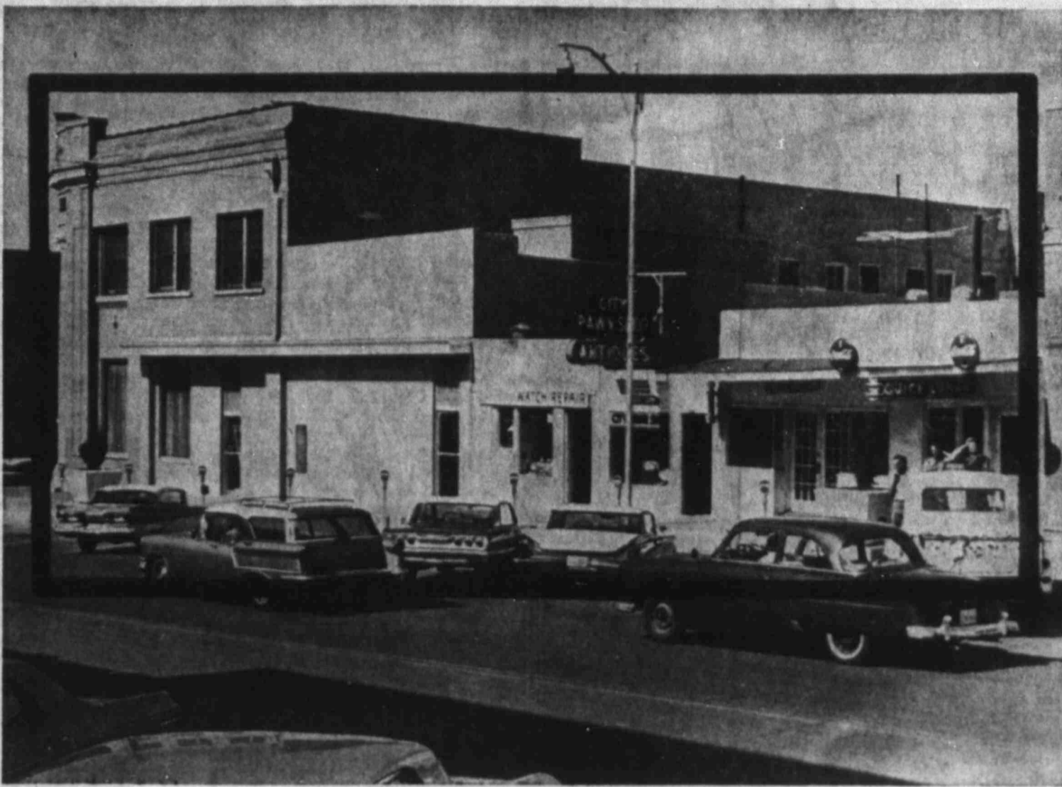
To Become Parking Lot
