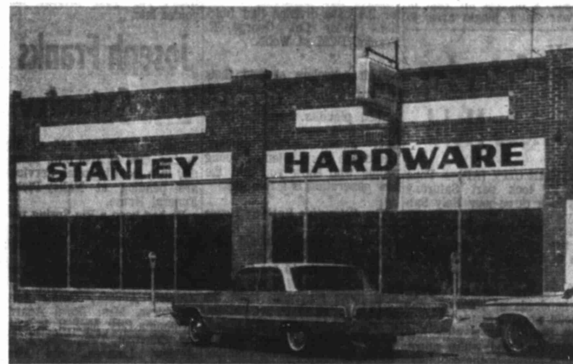
STANLEY HARDWARE PRESENTS NEW WEST FRONT Tinted glass placed on remodeled exterior
