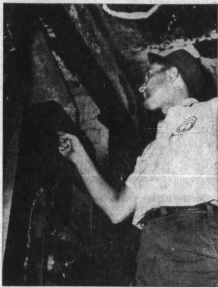
Shows Where Fire Started
