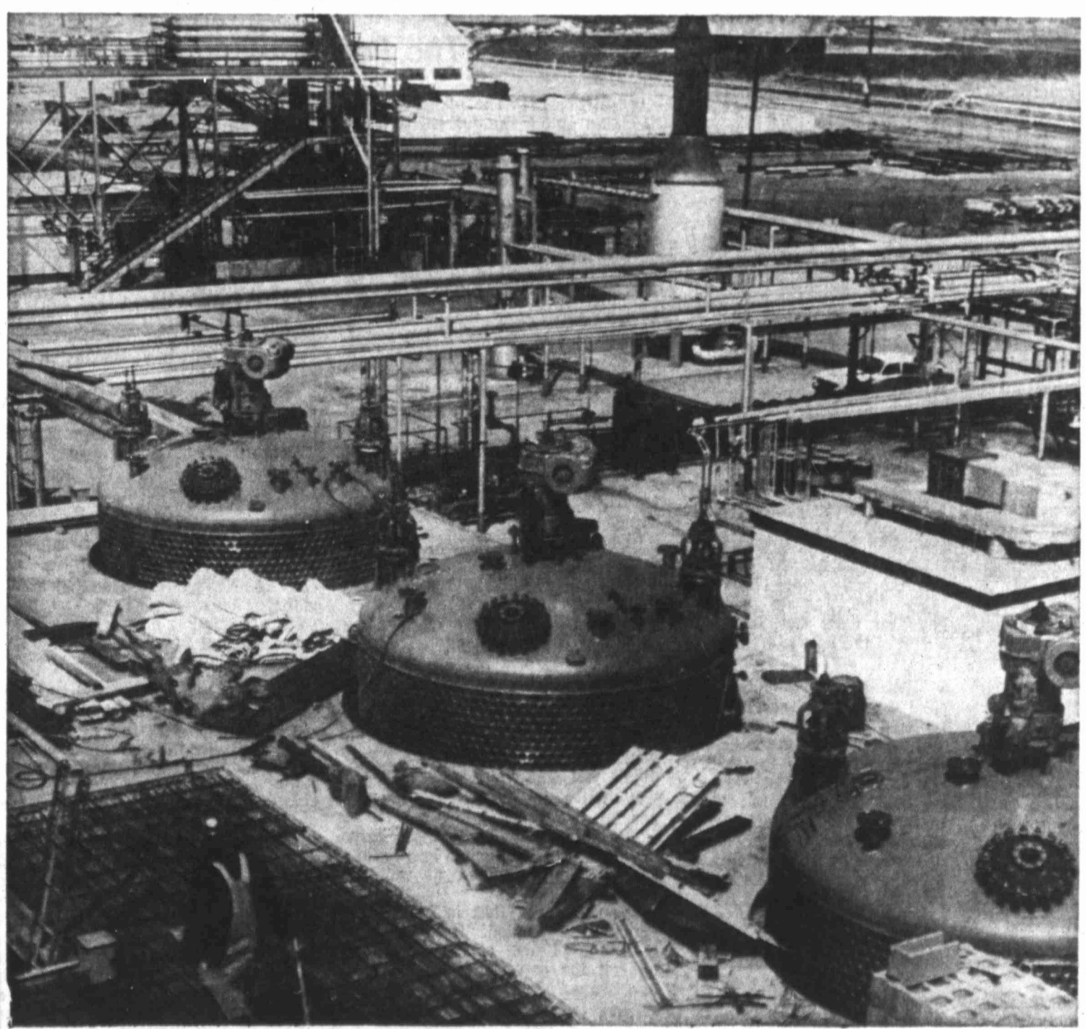
POLYSTYRENE EXPANSION AT COSDEN To be finished in mid-April
