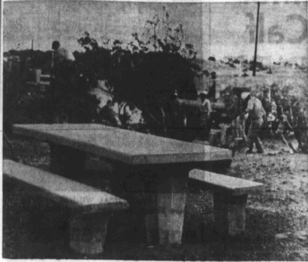
INSTALL CAMPSITE TABLES Ten Planned For Overnight Camp Area
