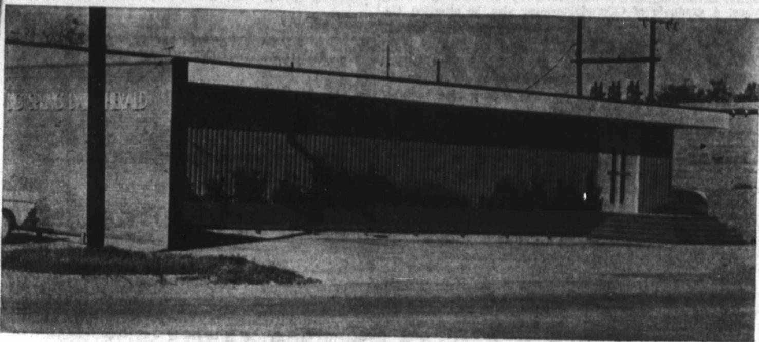
TODAY'S HERALD PLANT AT EIGHTH AND SCURRY Building, erected in 1956, houses staff of 60 persons
