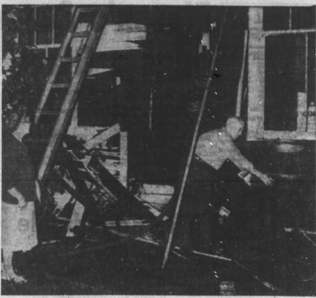
FIRE DAMAGE INSPECTED NEAR RIOT AREA Mr. and Mrs. John Krol look over ruins of golf course building
