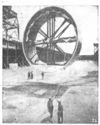
EASY DOES IT — Workmen, aided by hidden overhead crane, have no difficulty in guiding a 90-ton midsection of the sub Whale into place at Quincy, Mass., shipyard.
