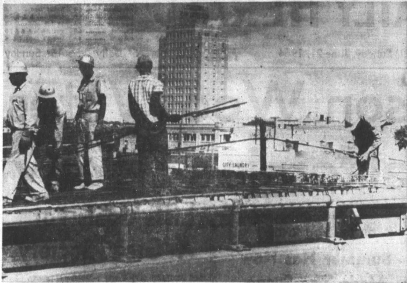
Steel Going In For Overpass Concrete
