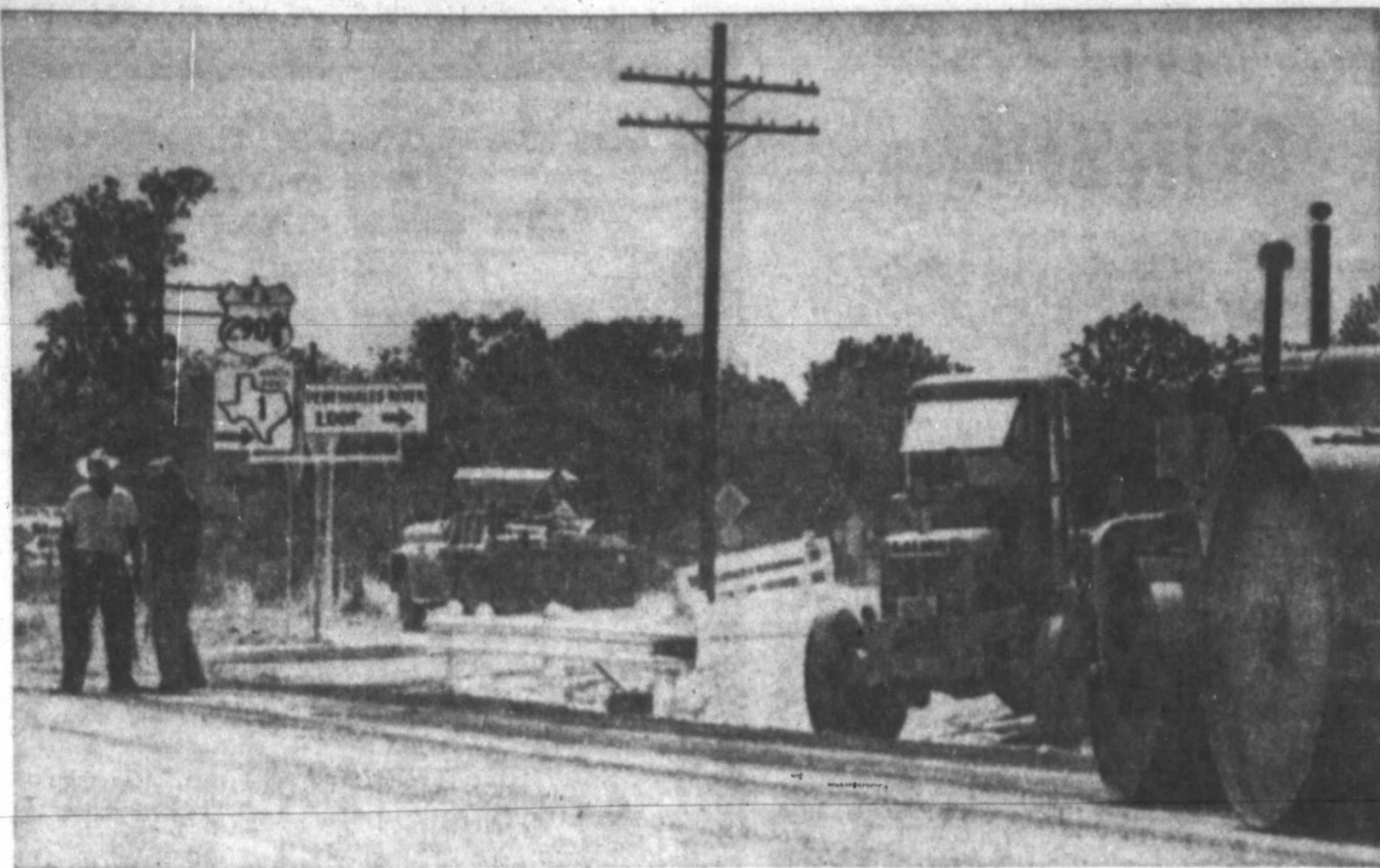
Work Nearing Completion On Ranch Road 1
