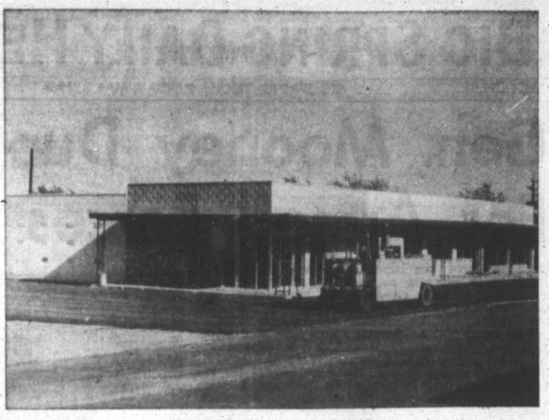
SOON READY FOR OPENING Six-unit Shopping Center on First Street east of bank
