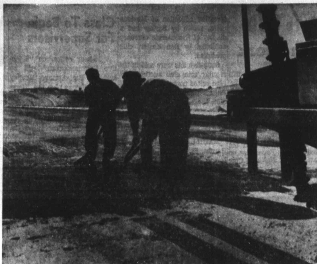
A BLACK RIBBON IS FORMING The priming base on the IS 20 by-pass route prelude to paving
