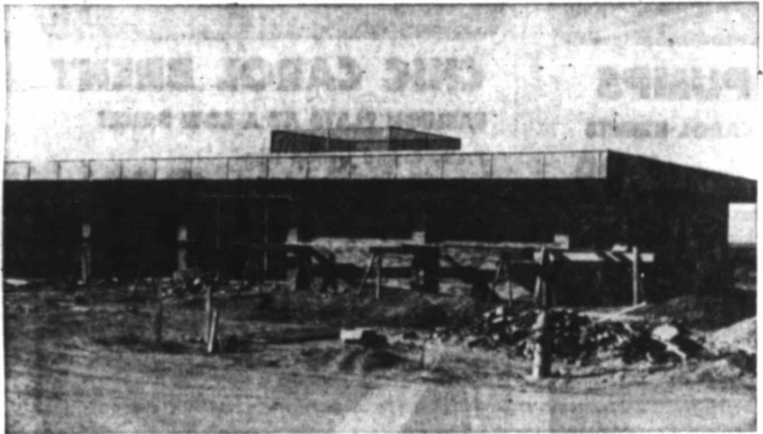
EXTERIOR COMPLETED At Airport Fire Station
