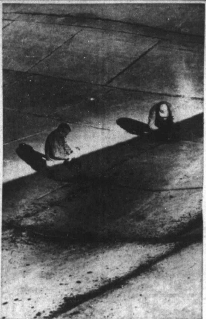
REPLACE CAULKING In 1,000,000 gallon storage tank
