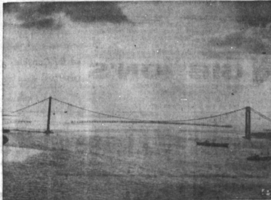
SPAN REACHES OUT —The roadway of Verrazano Narrows Bridge reaches out from towers near Brooklyn, left, and Staten Island. Nearing completion, the double-decked, two and a half mile span across the New York harbor will accommodate 12 lanes of traffic.
