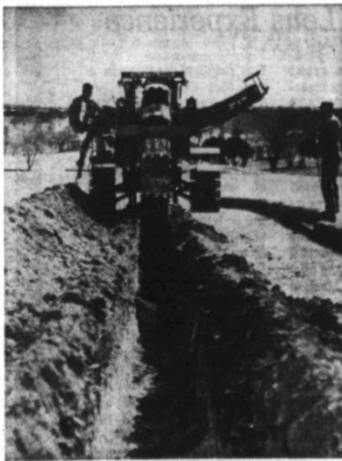
DIGS DITCHES For sprinkler system pipe
