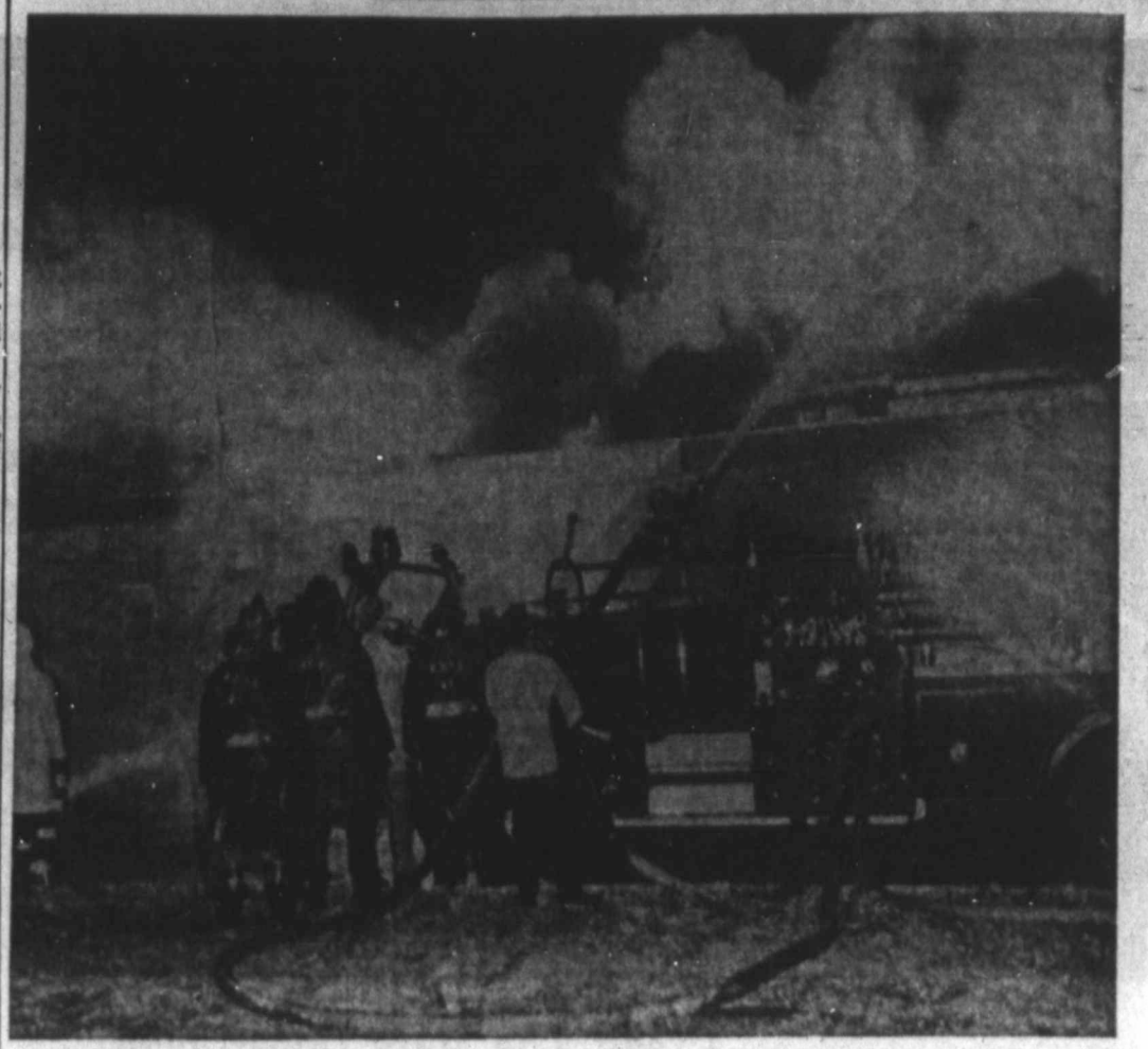
Fire Wrecks Discount Store Firemen pour water through the roof to fight flames which wrecked the Rink's discount bargain store in suburban Evendale early today. The loss to the block-sized brick building was estimated unofficially at more than $2 million.
