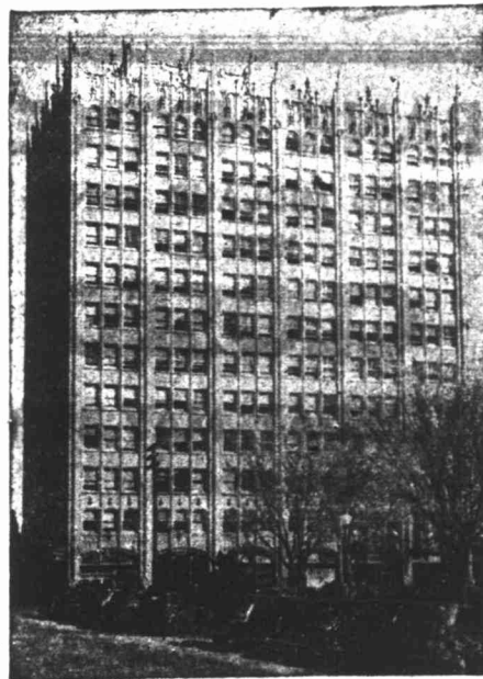
PETROLEUM BUILDING RALPH GEISLER, Bldg. Manager
