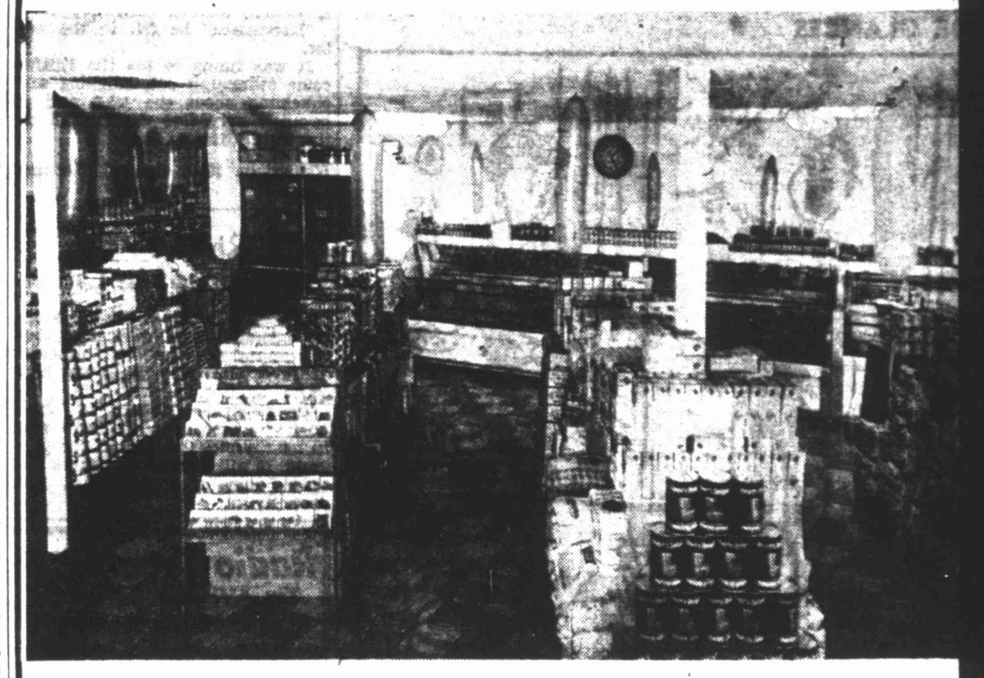
BROOKS GROCERY & MARKET NO. 2, Andrews Highway at Michigan Ave. Hours: 7:00 a.m. 'til 9:00 p.m.
