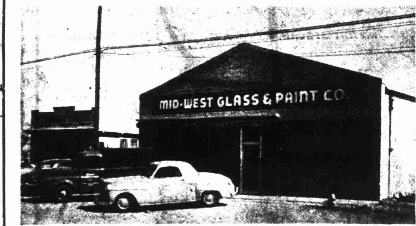
Shown above is the modern building that houses our up-to-date business. Inside this building you'll find glass for every purpose . . . paint for any use and metal and aluminum windows. You'll find courteous, helpful salespeople who will try their best to give you the kind of service you want. We invite your visit.
