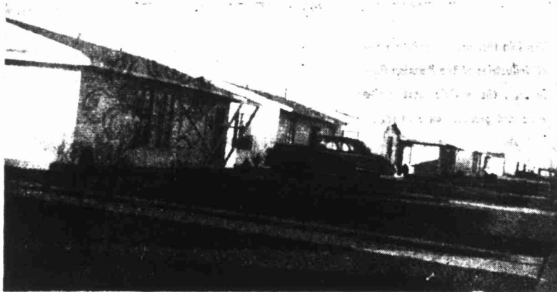
The Modern Paved Drive
