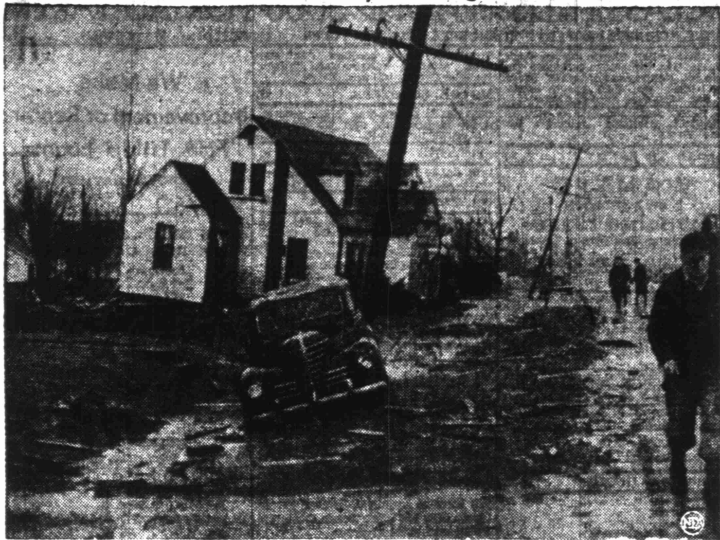
This house at Spanish Lake, Mo., was torn from its foundations and thrown into the gutter by a tornado which struck in Missouri and Illinois. The heavy hand of old man Winter swept across the Midwest, leaving freezing temperatures, tornadoes and flooding rains in its wake.
