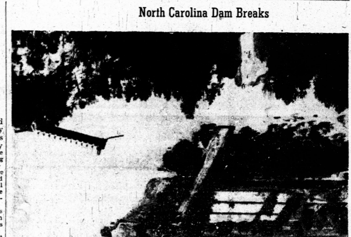
Millions of gallons of water rush through a break in the dam at Lake Brandt, the source of water for Greensboro, N. C. The dam broke from terrific pressure built up behind it by heavy rains of the last two weeks. Note the road which has been cut out by the swift-flowing water.
