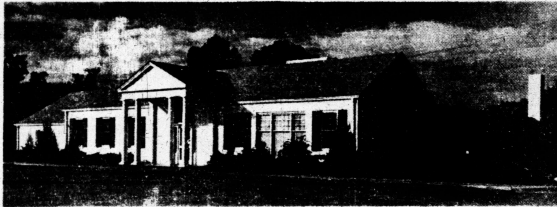
Construction will be started this week on the new plant of The Borden Company which will be located at the intersection of Missouri Street and West Highway 87 in Midland. The H. K. Ferguson Construction Company of Houston has the building contract, and A. Hays Town of Baton Rouge, La., and Wyatt C. Hedrick of Midland and Fert Worth are the architects. The new building and equipment will cost approximately $200,000. The Colonial-type structure will be of brick, painted white. It will have 11,000 square feet of floor space. When completed, the plant will be one of the most modern and best equipped in West Texas. H. B. Schauer is the firm's general manager here.
