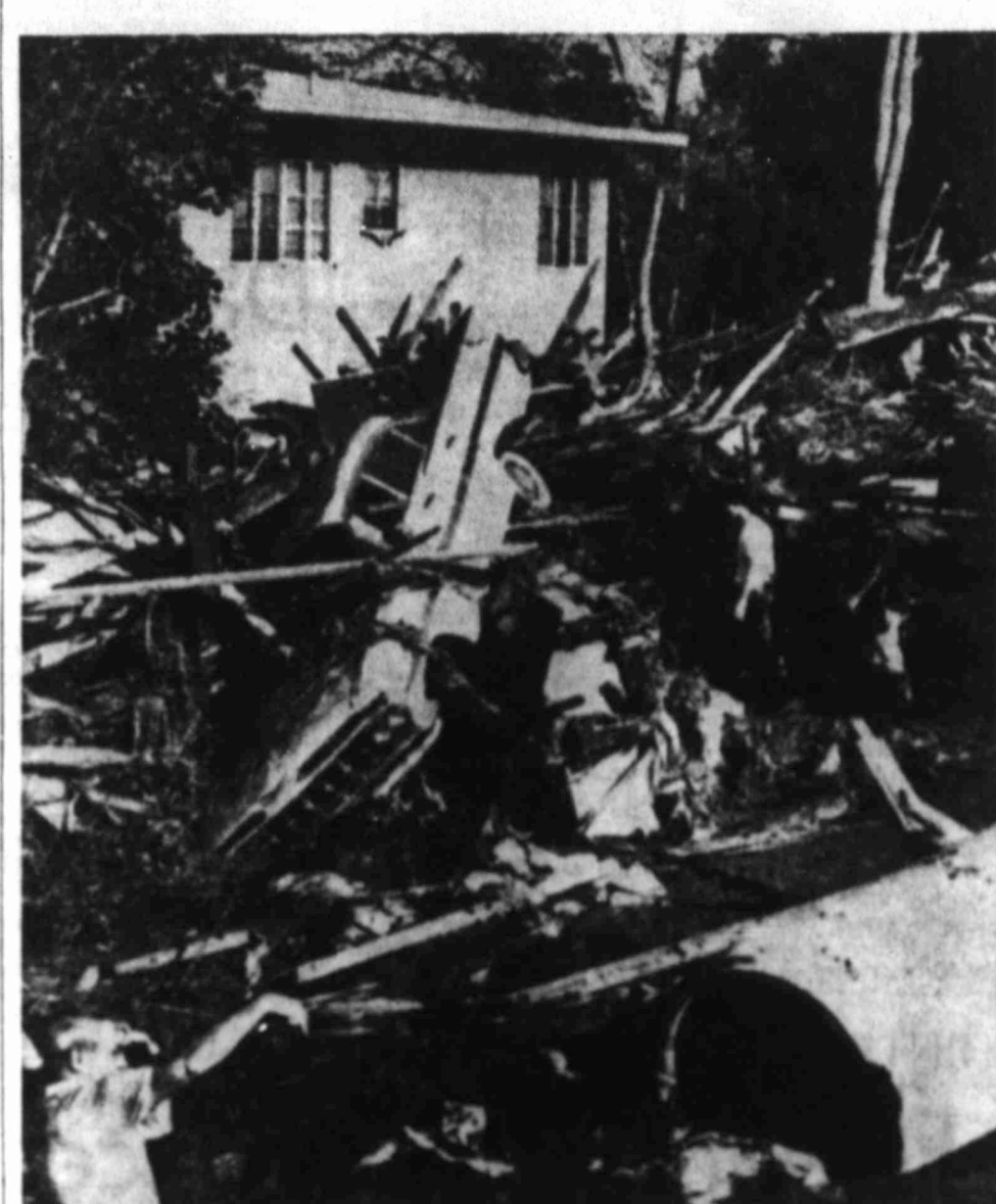
CARS, DEBRIS PILED UP BY FLOOD Los Angeles begins digging out from Saturday disaster
