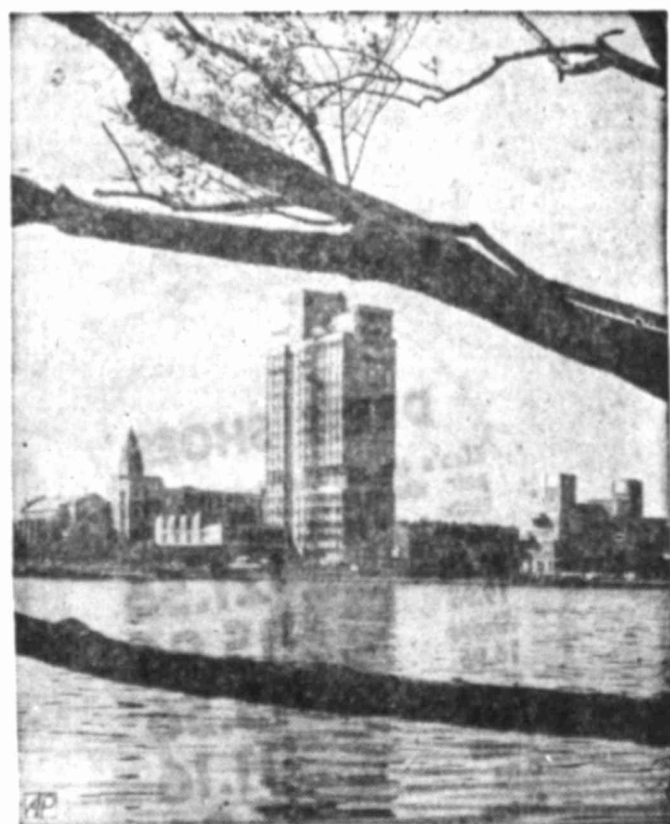
NEW LANDMARK —This 19-story structure is a newcomer to the bank of the Charles river in Boston. It will house Boston University's Schools of Law and Education.
