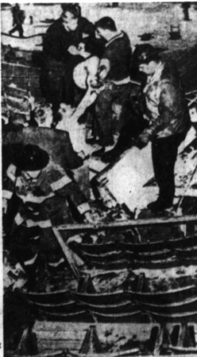
Victim Pulled From Debris
