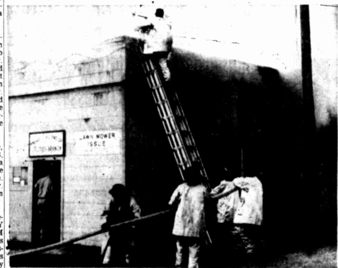
Fire Damages Building
