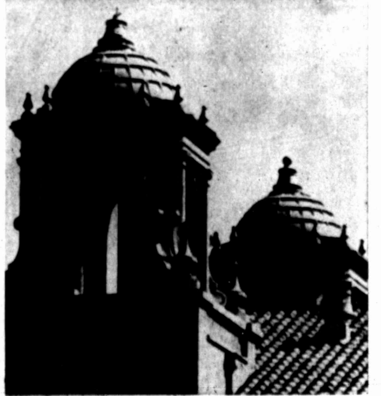
Lightning On The Ball. The ceramic tile ball, about 10 inches in diameter, on the east dome of the municipal auditorium, was shattered by lightning last night.
