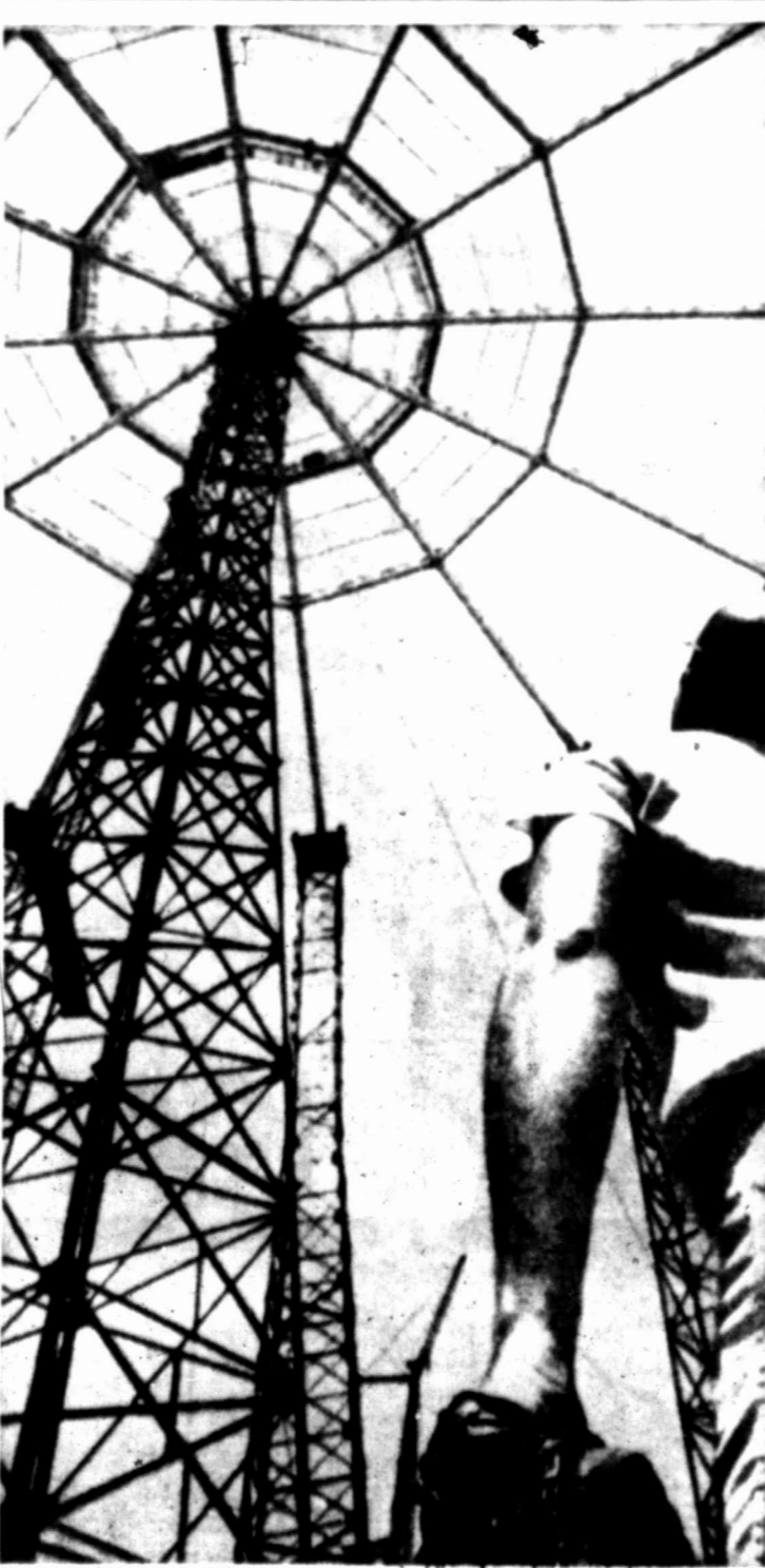
From The Top John Bateman, Houston catcher, looks up to the top of the steel works of the Houston domed stadium as he takes on some high dropped balls. Bateman took on the challenge to catch the high drops. A construction worker on the cat-walk of the web dropped the baseballs more than 200 feet to Bateman, who caught a few and missed a few. (AP WIREPHOTO.)
