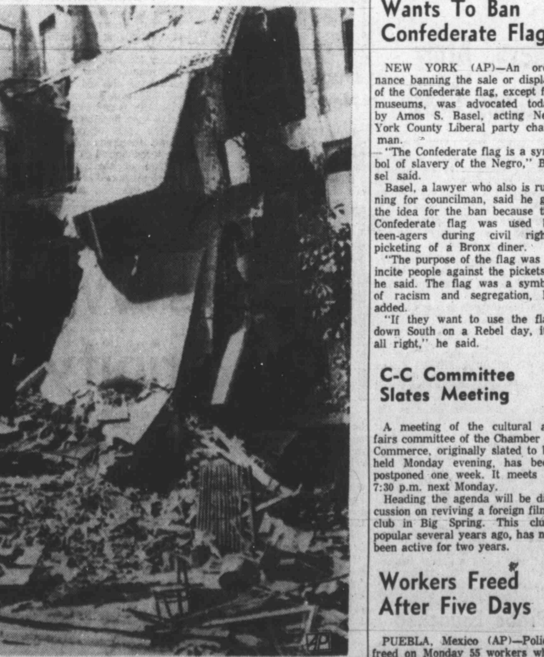
Quake-Shattered Structure In Skopje This is one of the many structures broken and ruined by an earthquake in Skopje, Yugoslavia in that country's worst national disaster in modern history. The upheaval of the earth cut down 90 per cent of the city's buildings and the remainder are being dynamited.
