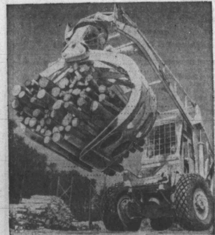
THE BIG LIFT —An American-built hydraulic lift carries a lumber load at chipboard factory in Thetford, England. It can handle 20 tons of lumber in 10 minutes.
