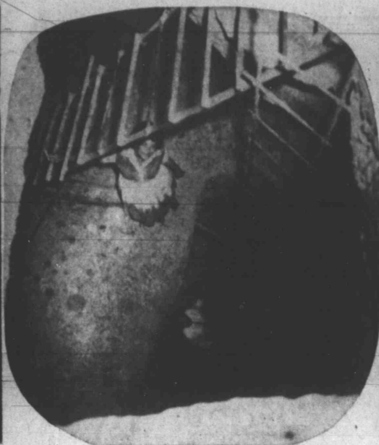
HAND-MADE WELL Dug with pick and shovel
