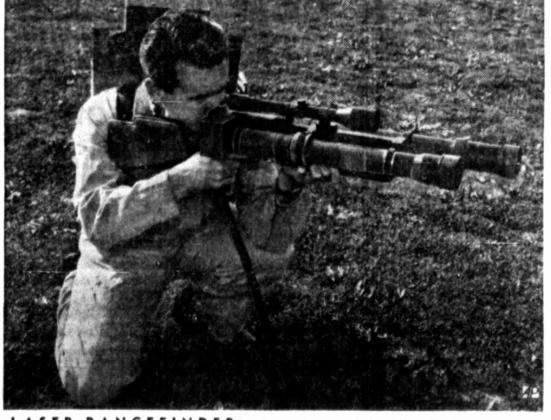
LASER RANGEFINDER - An engineer at Culver City, Calif., prepares to fire a laser light beam from barrel of Colidar used to pinpoint targets such as tanks. Telescope receives light reflected back and a timing circuit measures and indicates distance.
