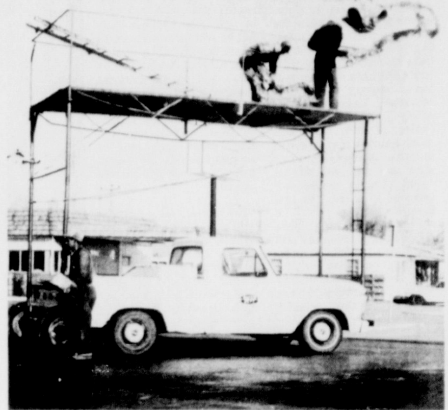
DECORATING TIME...City of Friona employees were busy earlier this week putting up the Christmas decorations down Main Street and Highway 60. The employees' job came at a brisk time, as
