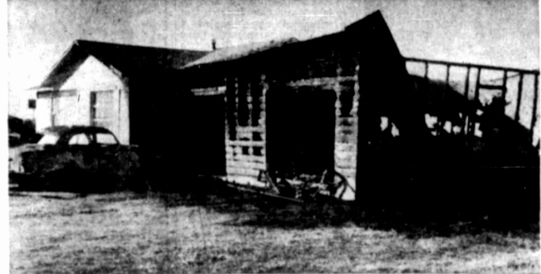
The Robert A. Fletcher home, on the Old San Angelo Highway, stood in partial ruins Tuesday morning following a flash fire that destroyed the garage and contents, including a car, Monday night. Big Spring firemen managed to cut the fire off between the garage and house but smoke and water did heavy damage to the interior and contents.
