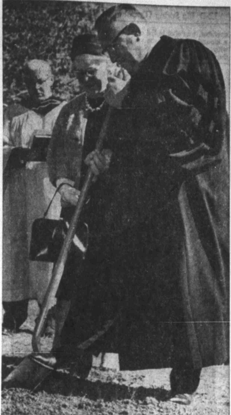
BREAKING GROUND ... for Presbyterian addition
