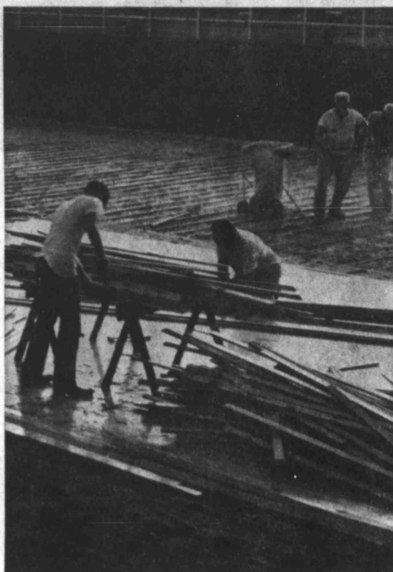
BRAND NEW FLOOR Repairs were many at the schools
