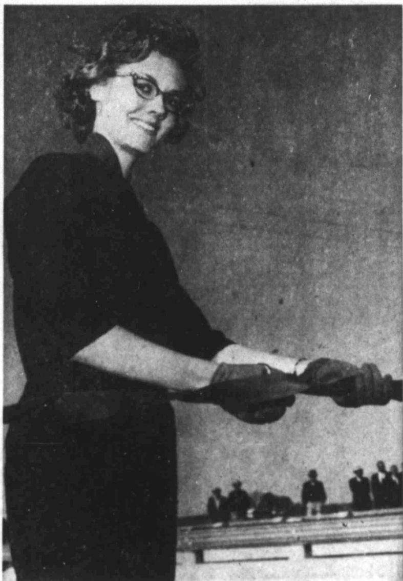
NEW BYPASS IS OPEN Janie Lee cuts the ribbon
