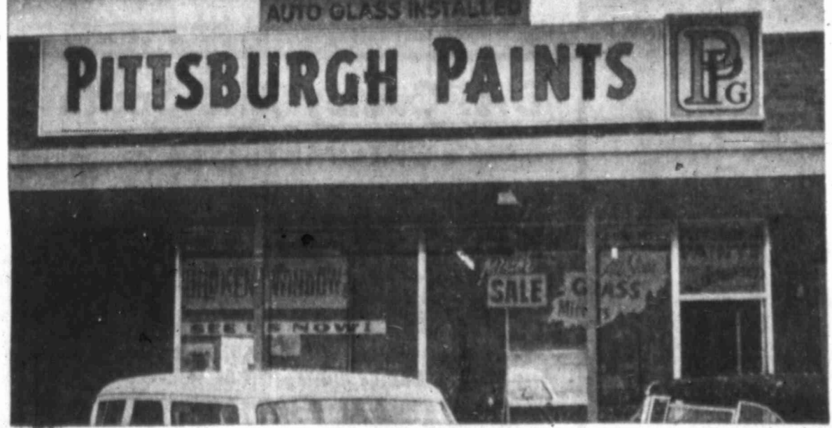
OPENS FIRST STORE HERE Featuring paint, glass, mirrors
